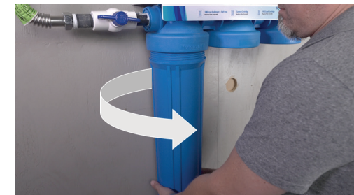
15) Insert the cartridge casing w/cartridge into it's designated position (Listed on Mounting Bracket) and thread by turning clockwise.
