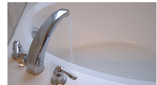
18) Restore the water to the home and allow water to flush through your new cartridges for 10 minutes.
