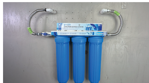
17) Repeat with each cartridge casing w/ cartridge. The cartridges are now replaced.
