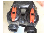
Bypass off, water flows through tank
