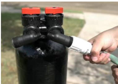
Carbon Filter Tank (CF)
